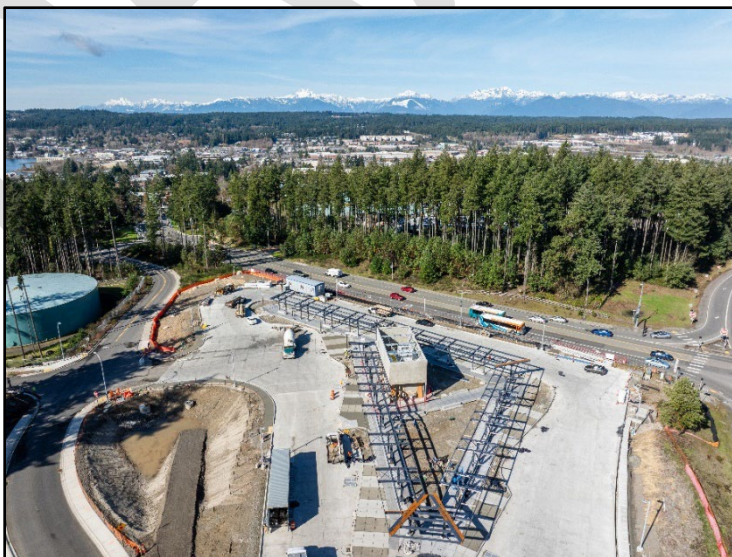
Construction progress on the new Silverdale Transit Center
